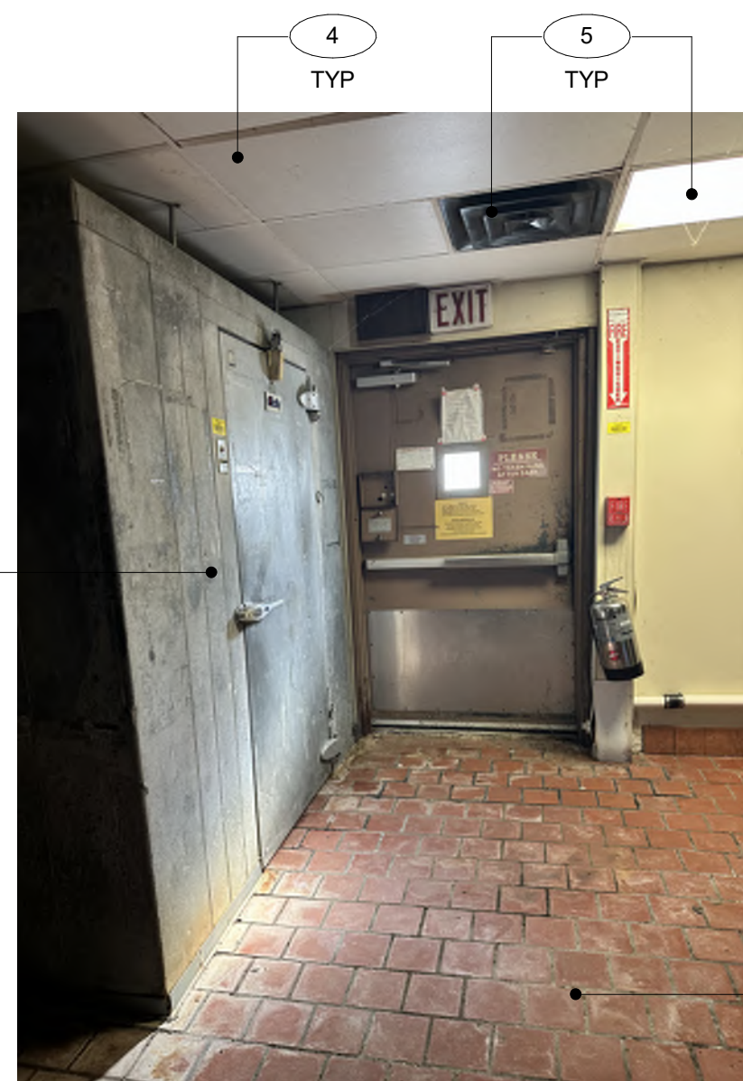
INTERIOR PHOTO-9: REAR ENTRY
