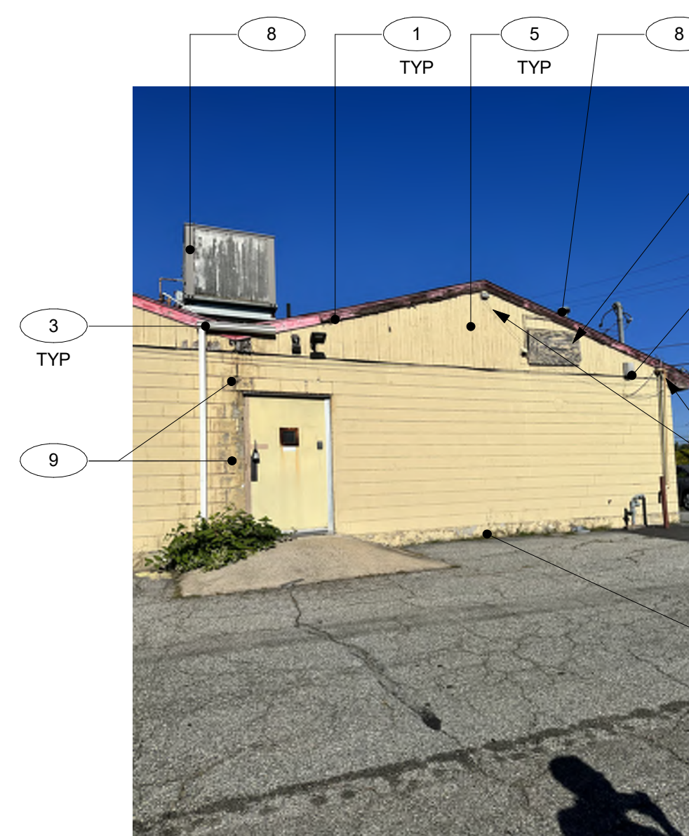
EXTERIOR PHOTO-7: EAST ELEVATION - RIGHT
