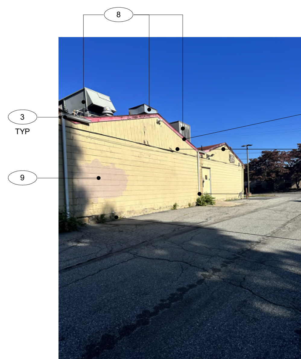
EXTERIOR PHOTO-6: EAST ELEVATION - CENTER
