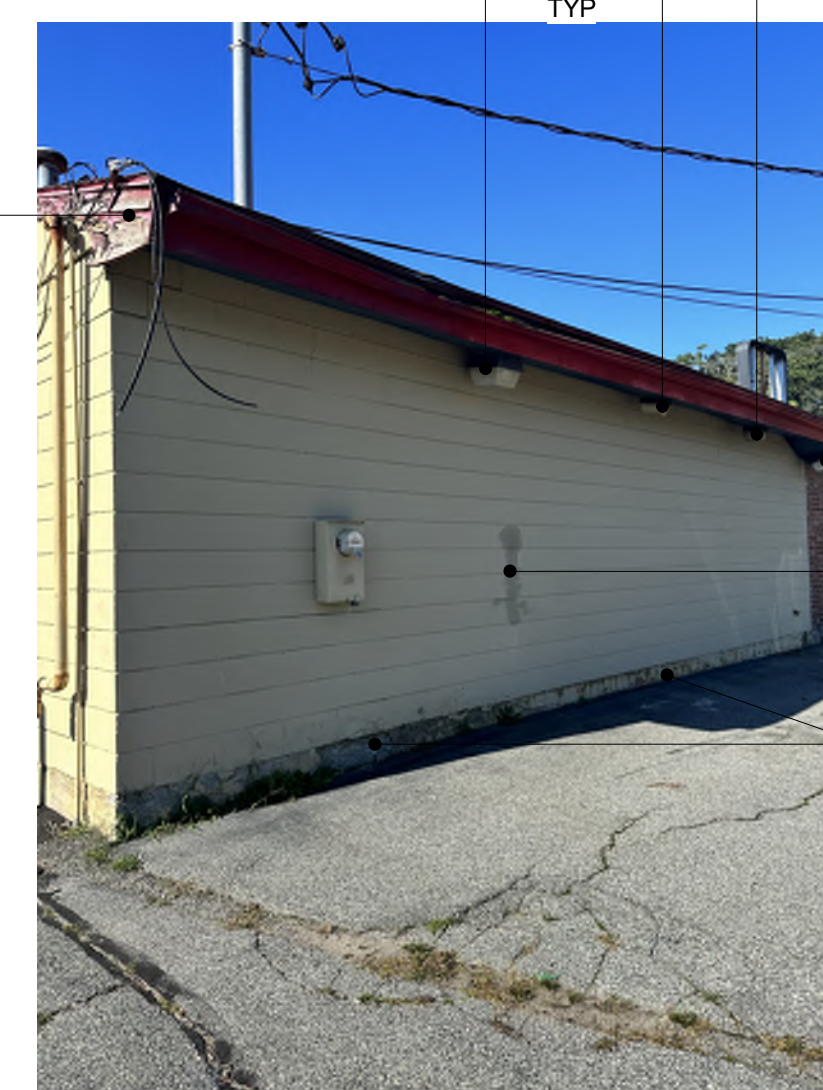
EXTERIOR PHOTO-8: NORTH ELEVATION
